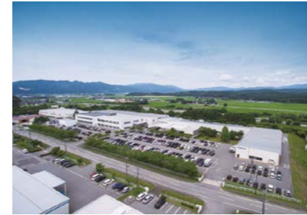
Head Plant, NIIGATA JAMCO CORPORATION
