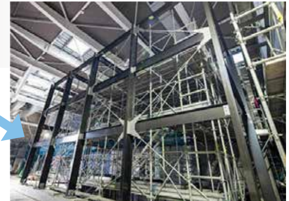
A vibration-proof and sound-insulating structure frame using CFRP
